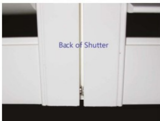
(2) Magnet keeping panels together
